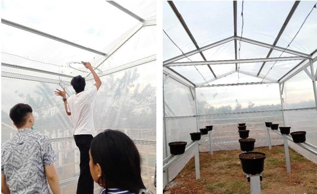
Proses Instalasi Misting Cooling System dan Finishing
